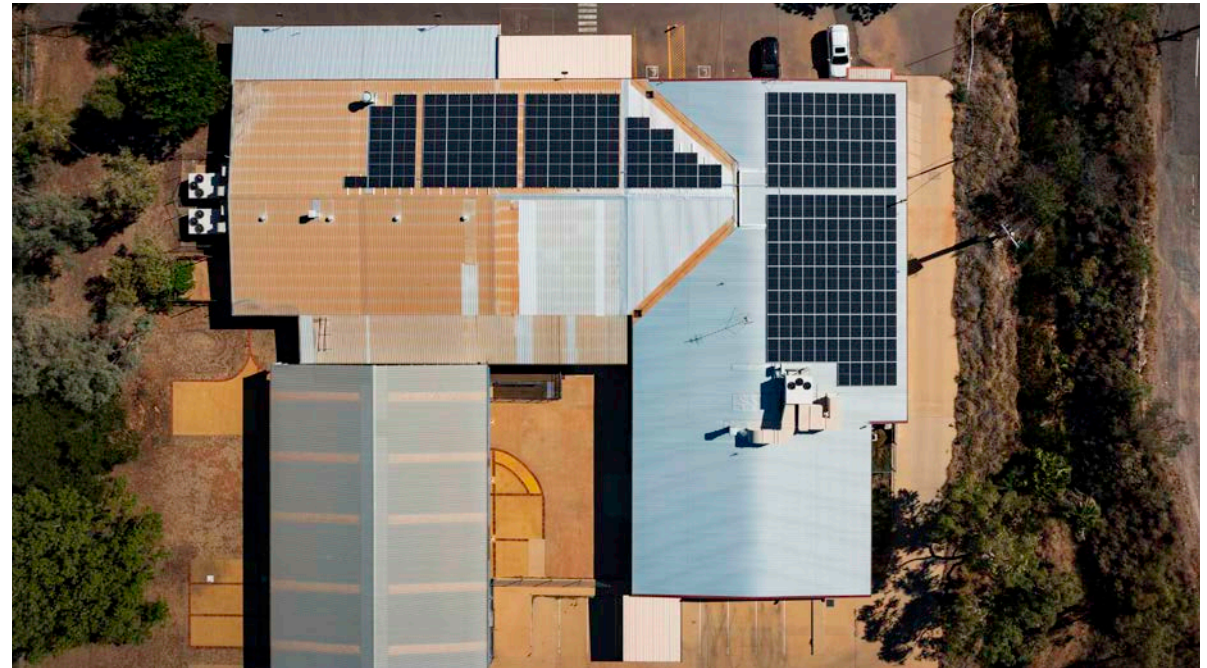
▲ New solar roof panels at Sonic HealthPlus Mt Isa GP Superclinic
